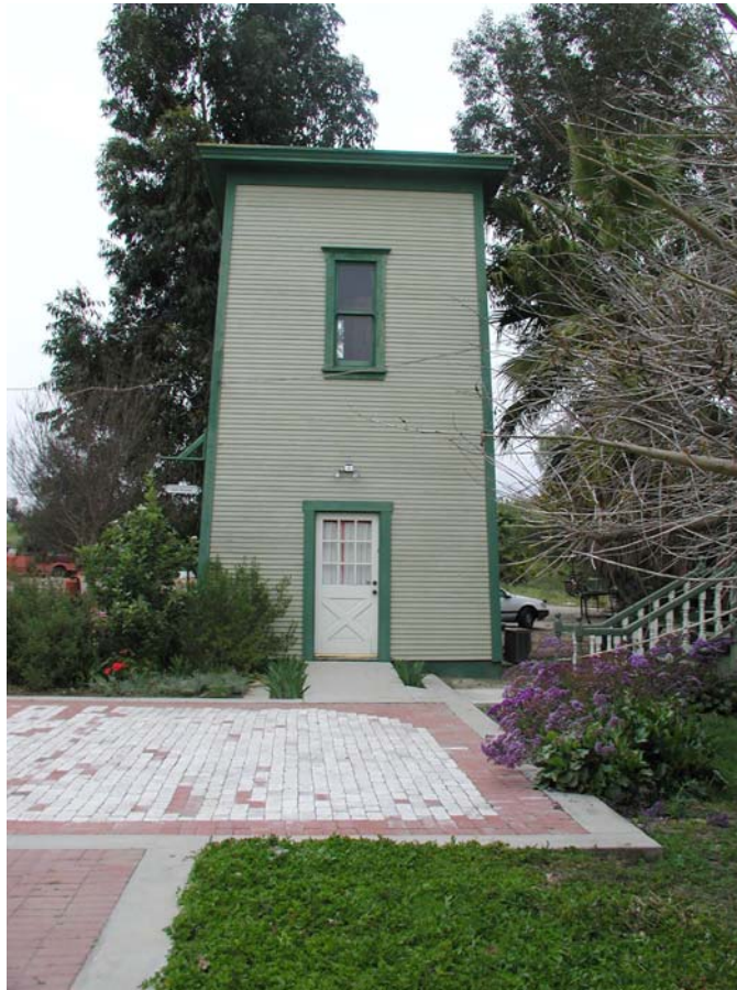
Maag Water Tower
