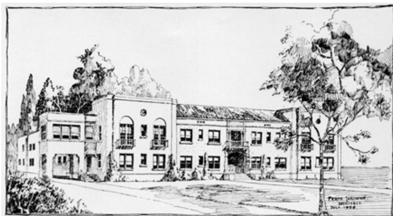
SANTA ANA VALLEY HOSPITAL—NEW UNIT
